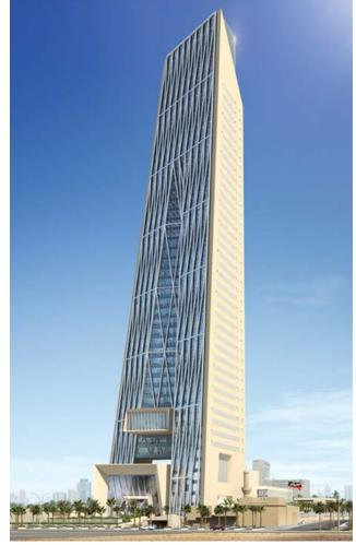
The two stone walls of the southern, city-facing tower reduce energy consumption by functioning as a heat sink to absorb the harsh Kuwaiti sun during the day and use the stored heat to keep away the cold at night.
